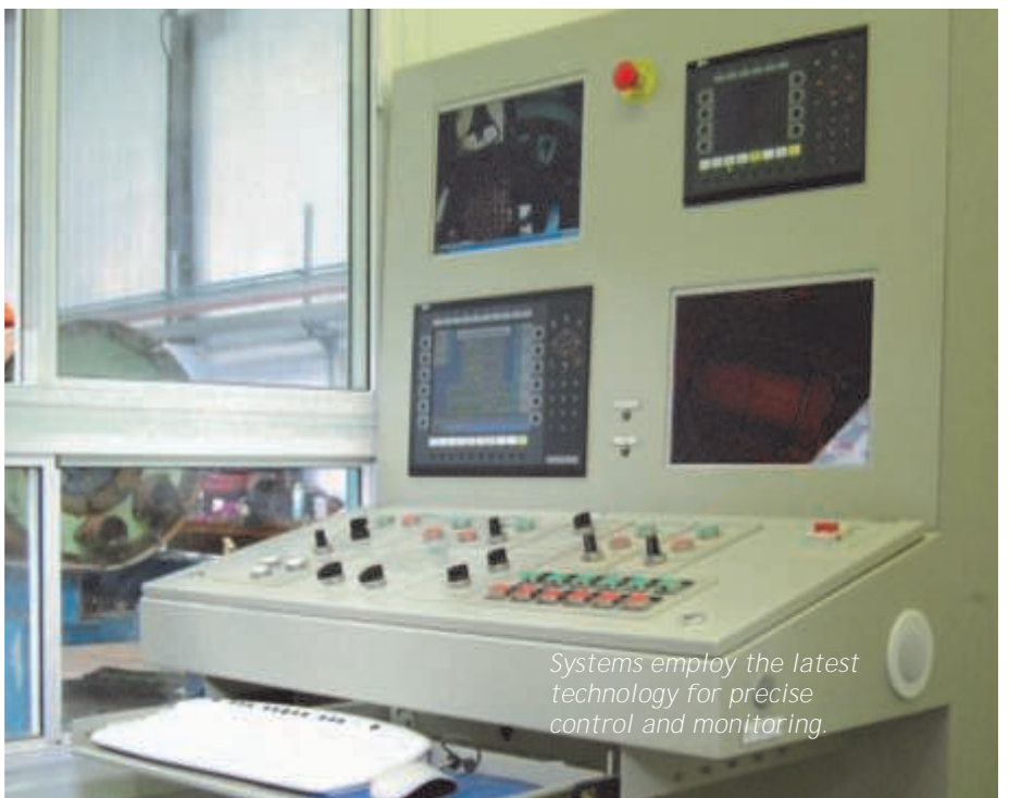
Operators have all controls to hand, and are able to see directly into the jacking shaft.
