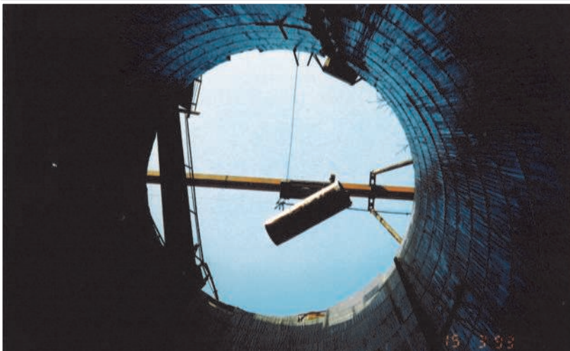
The machine descends into the shaft in Istanbul
