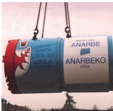
Lowering the machine into the shaft at Santa Catalina
