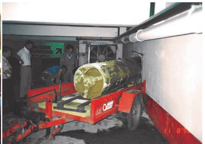
Machine recovery doesn't come any easier than driving the machine through a wall onto a trailer, like here at Le Mans!
